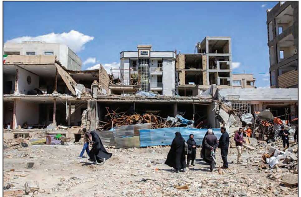
Residents in front of buildings damaged by airstrikes in Karaj, Iran, on April 3, 2026.
