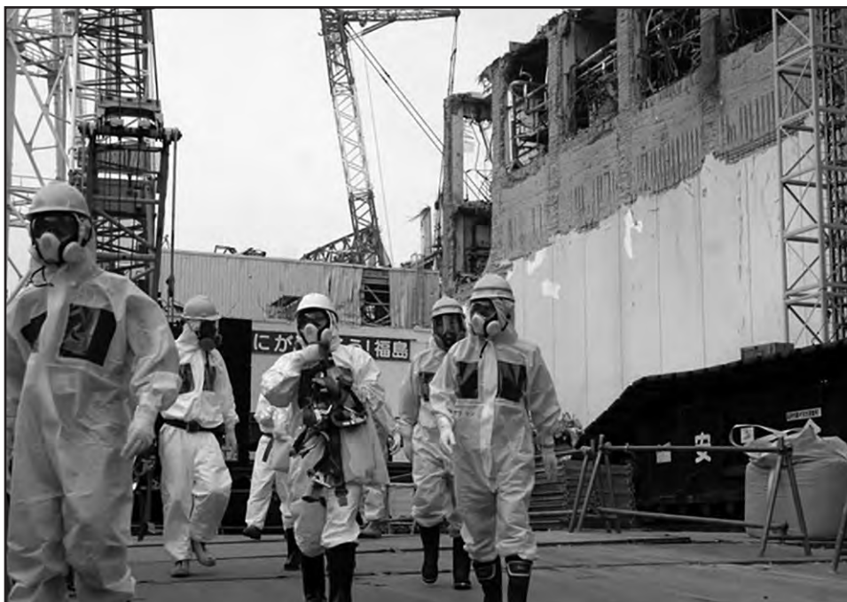
IAEA experts depart Unit 4 of TEPCO’s Fukushima Daiichi Nuclear Power Station on April 17, 2013 as part of a mission to review Japan’s plans to decommission the facility. Photo Credit: Greg Webb / IAEA
